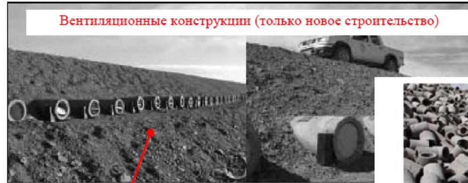
Figure 4: Ventiduct Embankment with shutters
